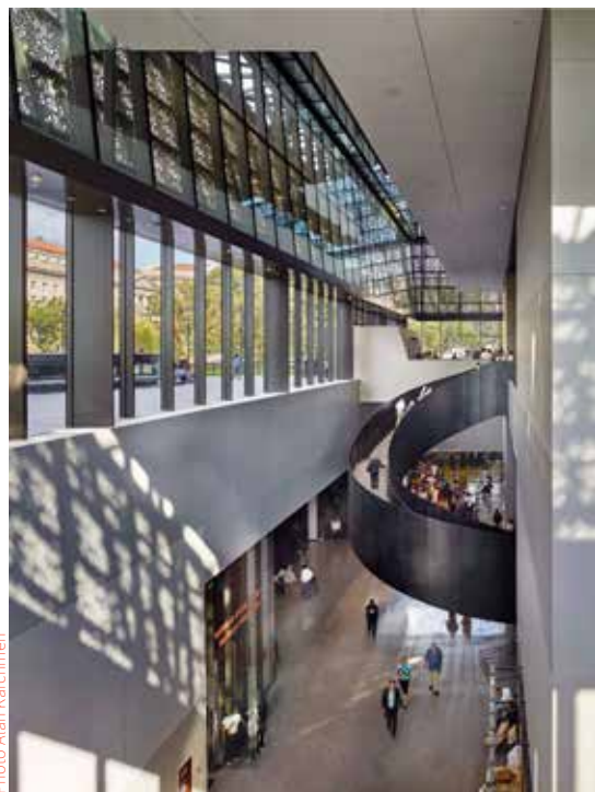
独立支撑的柯尔顿钢制楼梯/Self-supporting Corten steel stair
